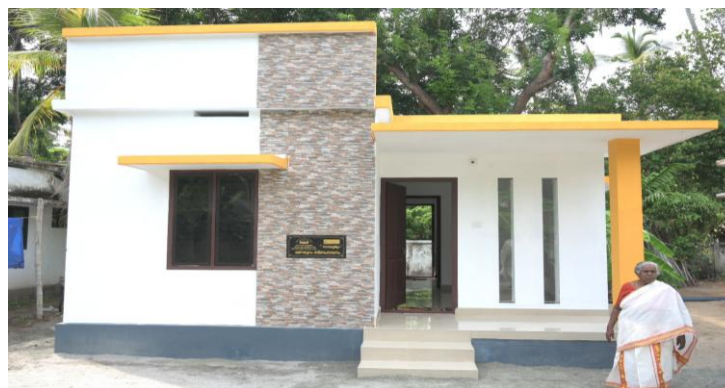
Provided a home to Ms. Santha Narayanankutty of Sayujyam under the Sayujyam housing initiative, which has earlier delivered 13 new houses and completed 3 renovations.
